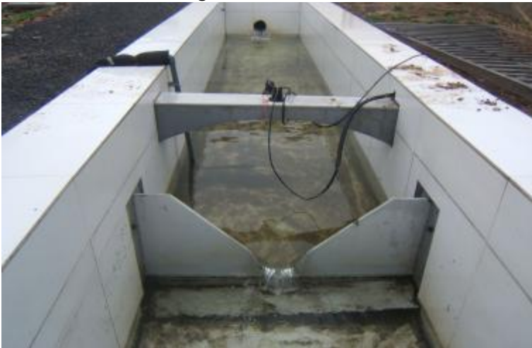
Figure 4.3.1 Triangular Weir
